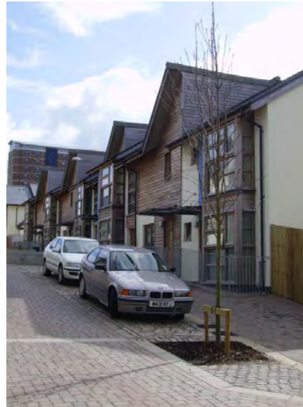
Fig 5.21 Well-designed on street parking can make a positive contribution to the street scene.
