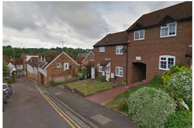
Fig 5.13 The existing homes on the nearby Chapel Street step down the steep hill and provide level access for each dwelling. Front gardens are terraced with the levels of the road.
