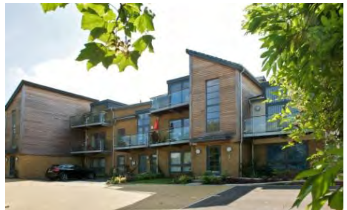
Fig 5.17 Although more modern in style than other examples the articulation of this facade provides opportunities for balconies with privacy from overlooking.
