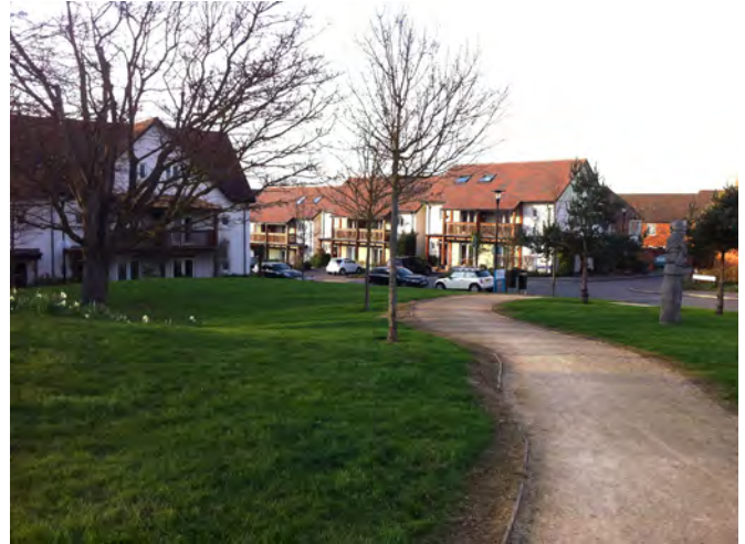
Fig 5.12 The buildings in this example step down with the topography of the site and the open space has been designed to incorporate existing levels and features.
