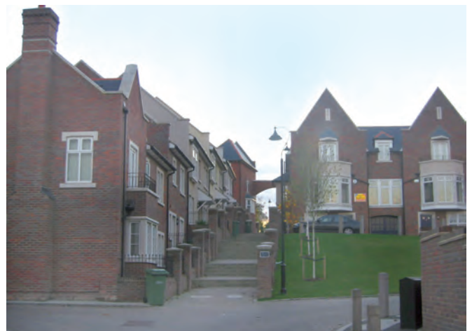
Fig 5.14 The buildings at Greenhithe step down a steep slope creating an interesting pattern of roofs, whilst also allowing level access to new homes.
