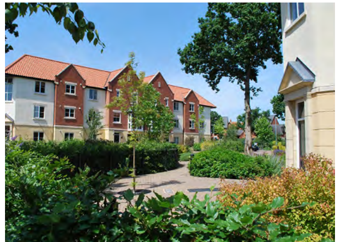
Fig 5.16 The articulation of the elevation of these flats help to break down its overall massing and is also in keeping with the surrounding housing development.
