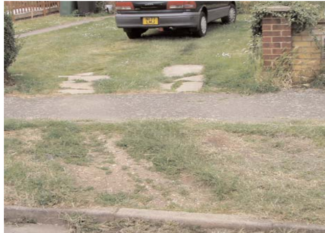
Grass verges have been damaged by cars.
