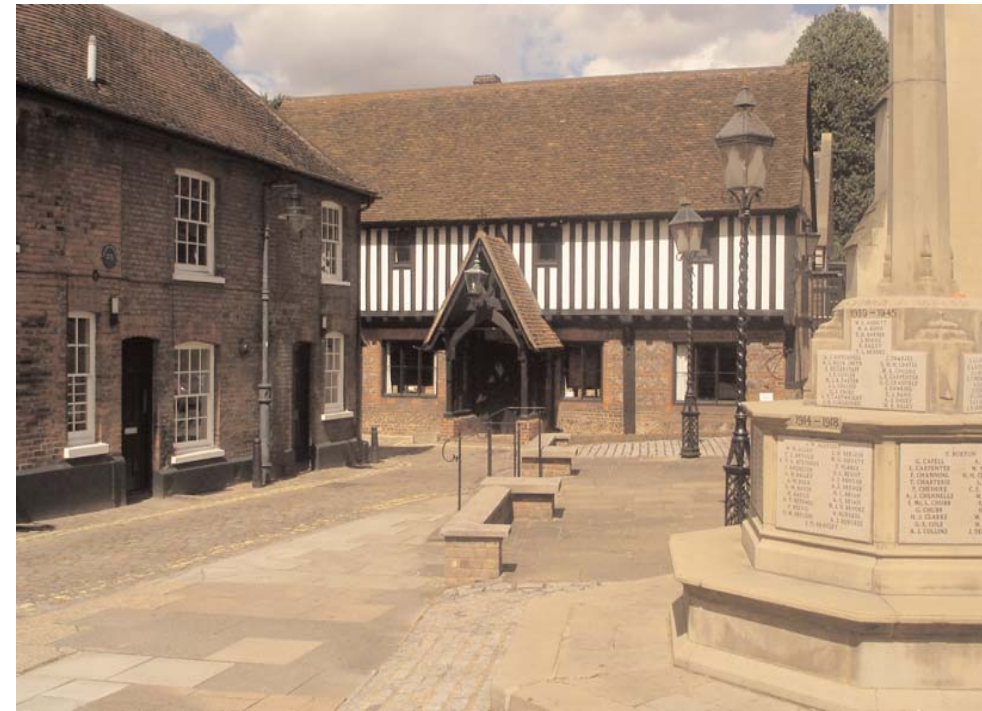
The upper floor of the Court House is of 16th century timber framing and the ground floor of knapped flint and red brick were added in the late 19th century by William Butterfield.
