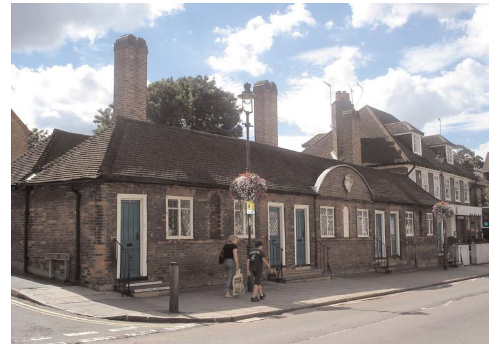
The Sayers Almshouses, built to house poor elderly widows, were the gift of the widow of John Sayers, Charles II's chef.
