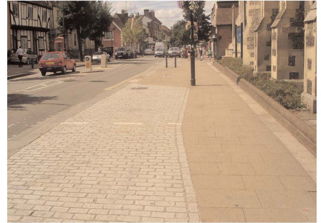
The parking bays have discrete paving at the level of the pavement, not the street bed.
