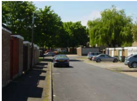
Grovehill in Hemel Hempstead has some design flaws, such as pedestrian unfriendly alleyways (top) and areas dominated by tarmac, car parking and garages (above). These sorts of features need to be avoided in the design of the new neighbourhoods.
