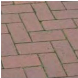
Concrete red coloured bricks arranged in a fishbone pattern
