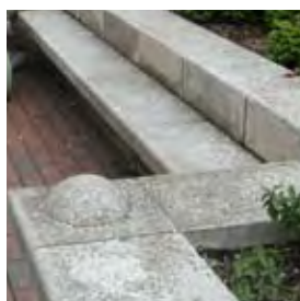
Pre-cast concrete used for planters, integrated seating steps and fountain bases
