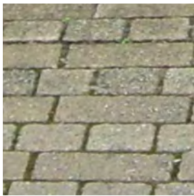
Rows of grey concrete bricks arranged in rows of full and half sized bricks
