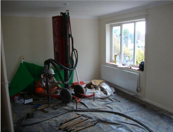
This image above shows our Dynamic Probing rig working inside a vacant property on Pond Rd – this has allowed us to refine our methodology for gaining access if we are required to undertake validation within a property. We will be working with Hyder to avoid validation works within properties wherever possible.
