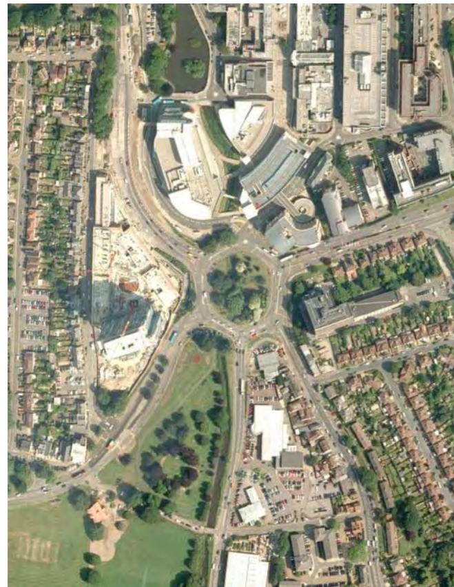
Aerial view of the Plough Roundabout
