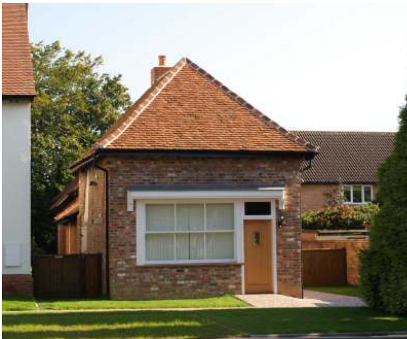
Although just outside the Conservation Area, the old Butchers Shop at New Hall illustrates how sympathetic repairs can give new life to a historic building whilst retaining its character
