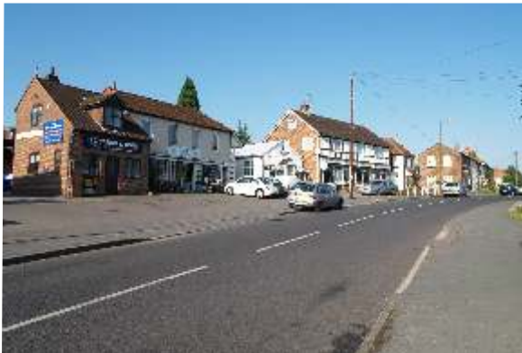
The hard surfacing and lack of planting in this part of the High Street creates a harsh urban landscape
