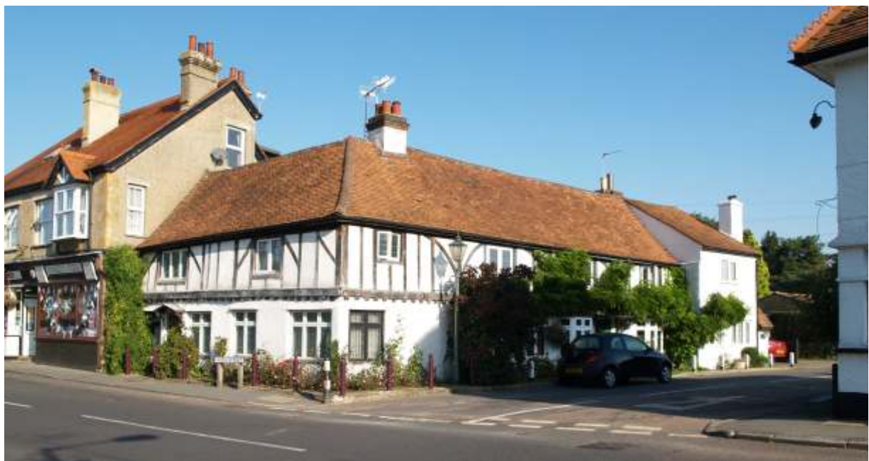
Nos. 83 High Street and Nos 1-3 Church Street are locally listed buildings
