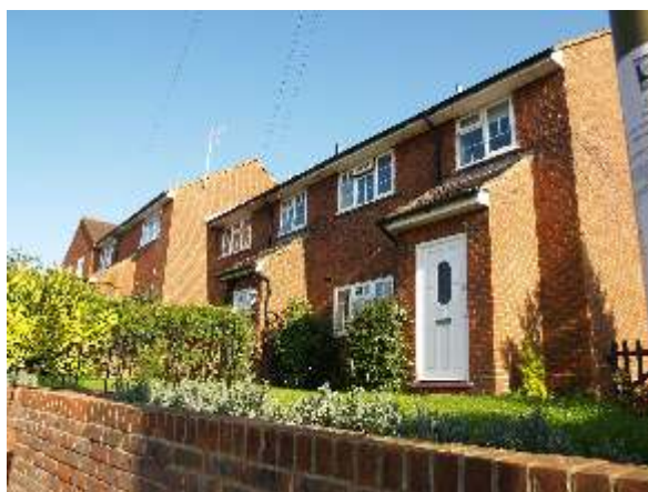
C20th housing infill in the High Street
