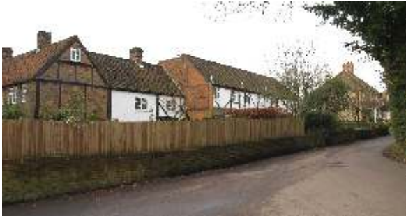
The poor materials, muddled fenestration and high close-boarded fence of Lychgate Cottages, together with the crown roof, false framing and unsightly flues of the C20th range facing Vicarage Lane illustrate how piecemeal alterations and additions can erode the character of the Conservation Area
