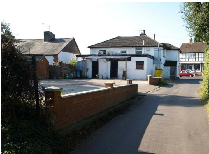
Inappropriate boundary treatment creates a harsh edge, unrelieved by any planting
