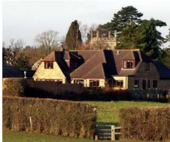
Though just outside the boundary of the Conservation Area, the extensions and awkward handling of the roofscape to this house and its boundary walls jar with its rural setting and block views of the Church
