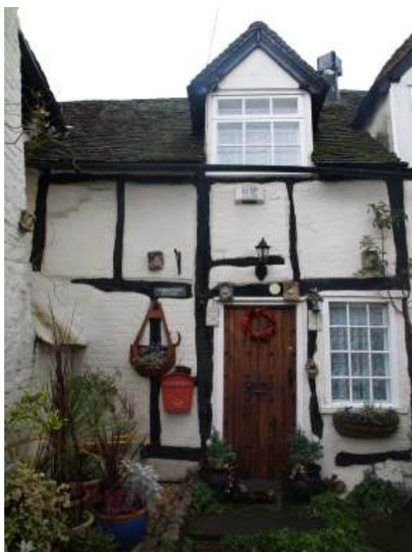
No. 84 High Street, a former open hall house with large panelled timber framing
