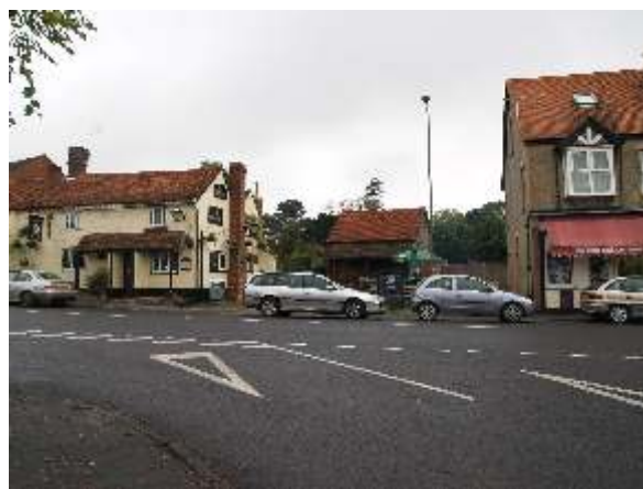
Spaces between buildings are as important as the buildings themselves. Note also the contribution the ancillary outbuilding makes to the streetscene.
