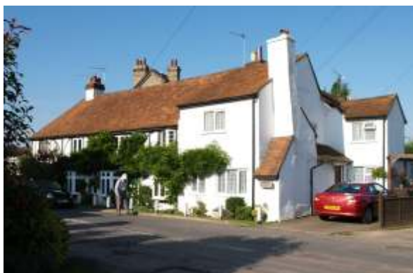
Tiled roofing predominates in the Conservation Area. Note also the tiled offsets to the chimney stack (Nos. 1-3 Church Street)
