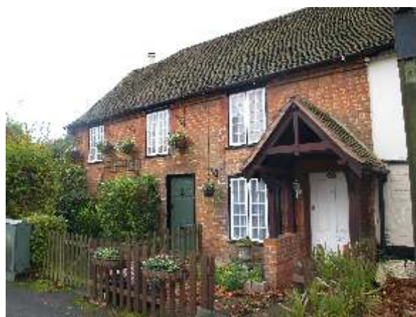
The timber framing of Nos. 106 & 108 High Street was encased in brick in the C18th
