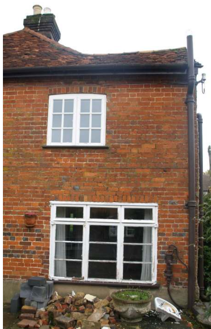
Much altered brick walling to rear of Yew Tree, Incorporating some burnt headers
