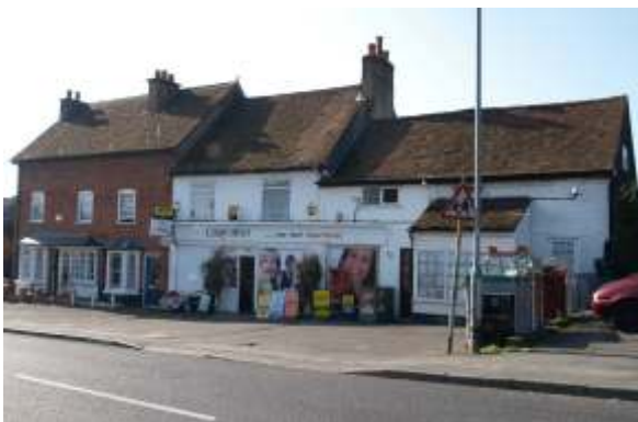
Graduated tiled roofs create a pleasant hierarchy, undermined by the poor shop front, signage and hard landscaping
