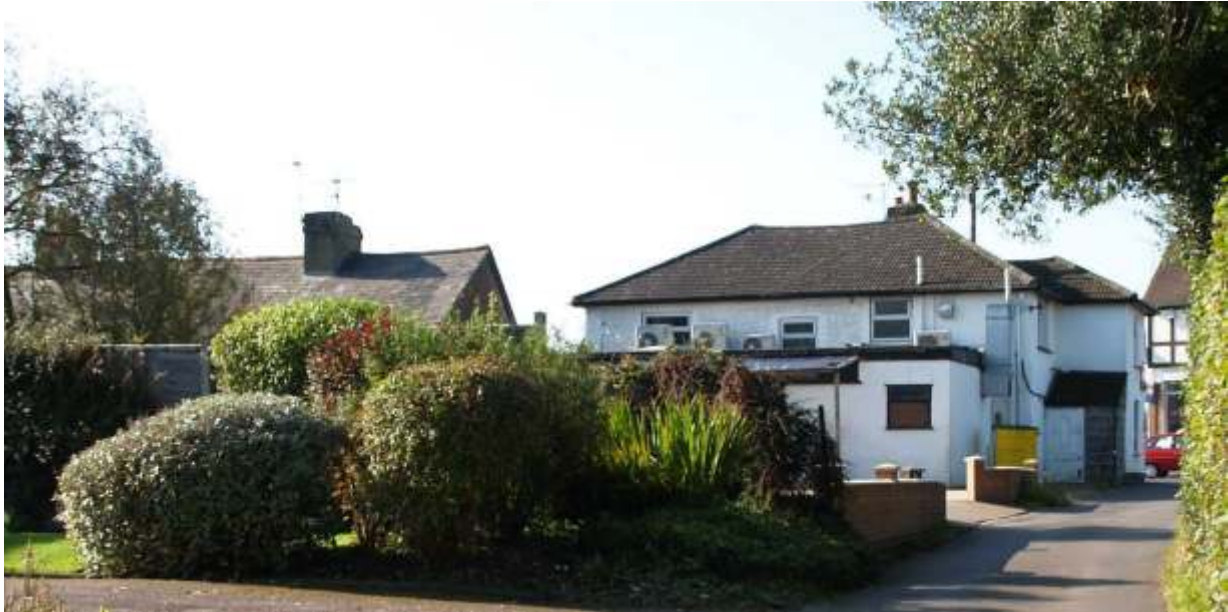
Slate was used from c.1800 in Bovington. Pitches tend to be flatter. The cottages to the left are slated at the rear, but tiled to their steeper-pitched High Street frontages
