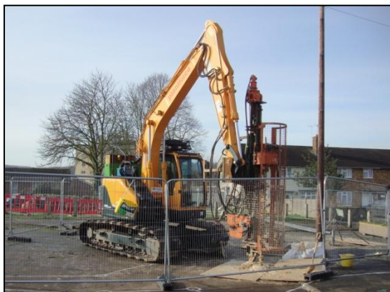
Excavator mounted drilling mast in operation on Highbarns
