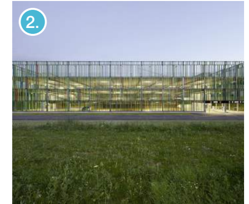
Artificial green facade
