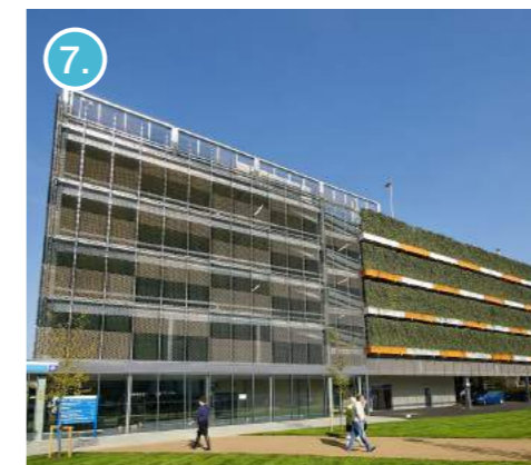
Soft-cladding - wide balustrades to allow grass to coat the exterior of the frame
