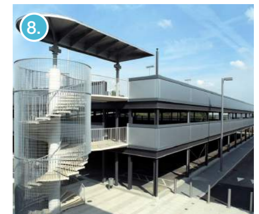
Steel-framed and column free
