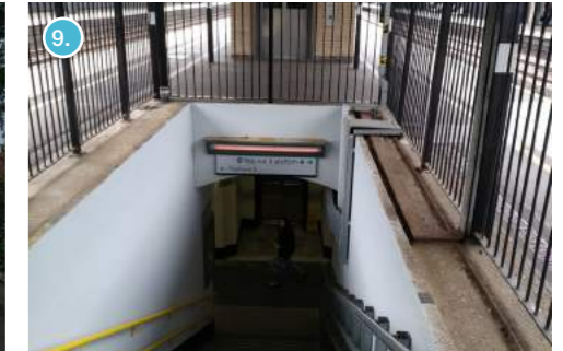
9. Stepped access to platform level
