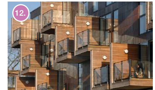
12. Balconies/winter gardens facing the moors
