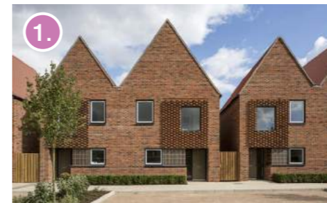
1. Pitched roof - varied and interesting roofscape
